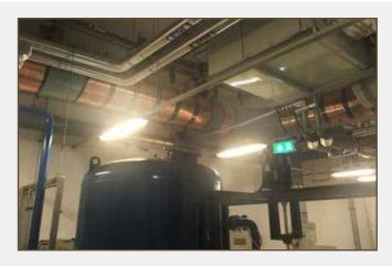
Mineral Descalers are installed on the condenser main return pipes; supporting 7 cooling towers.
